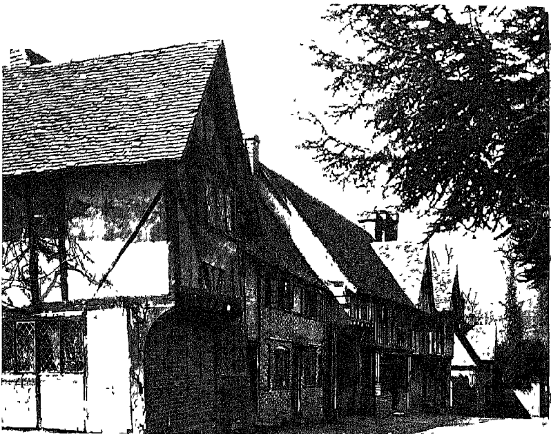
§ 152 Tudor cottages, Chiddingstone, Kent Note the use of brick between the timber uprights
